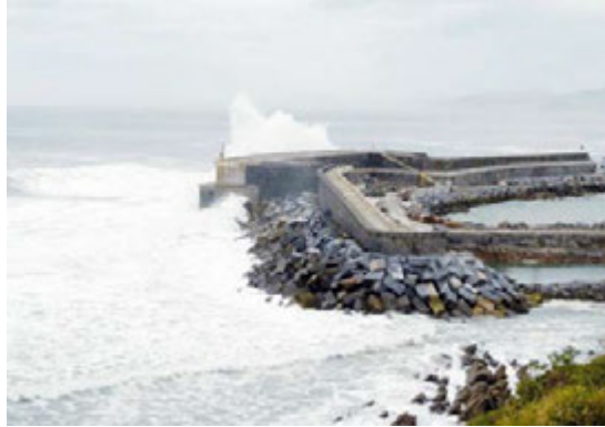
Figure 8.2. Mutriku, Spain, oscillating-water-column-breakwater integration. Source: obs/Voith GmbH
